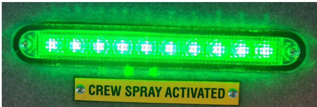
Figure 4.179 - Deluge Activation and Pressure Indicators
